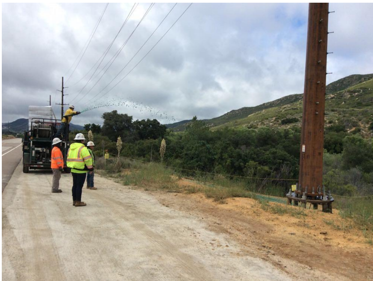
Photo 6: Application of hydro-mulch for restoring the native habitat was observed at Pole Z40512 (TL 629C) in accordance with MM BIO-4. An archaeological monitor was also observed monitoring the activities in accordance with the HPMP, APM CUL-04, and MM CUL-1.
